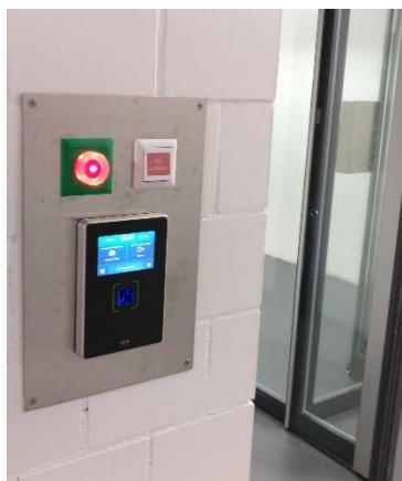
After placing the goods inside the lock, pass the man-trap and get the material from inside out of the goods lock (authorization via fingerprint and finally close the door with the button “Türe schliessen”).
